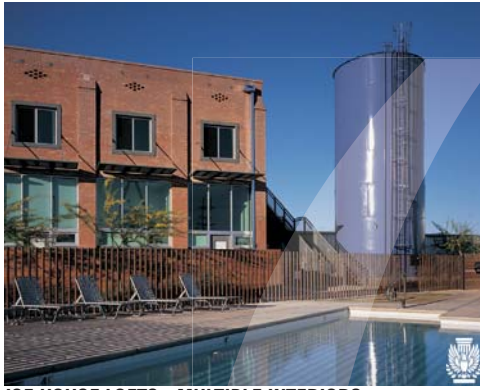
ICE HOUSE LOFTS - MULTIPLE INTERIORS (Rob Paulus Architects Ltd.)
